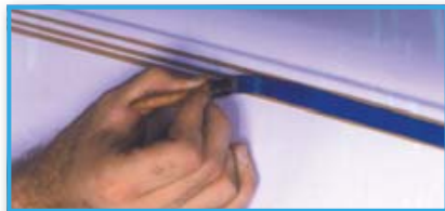
Paint over the stencil.
