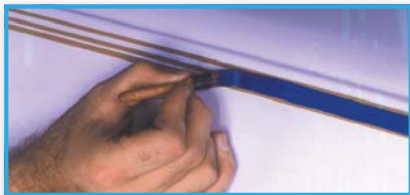
Paint over the stencil.
