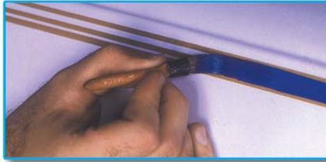
Paint over the stencil.
